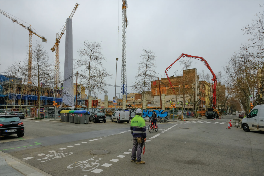
FIGURE 27 A smokestack wrapped in plastic in the Poblenu neighborhood, protecting the structure as the former industrial site is converted into a large, market-rate housing complex, 2021.
