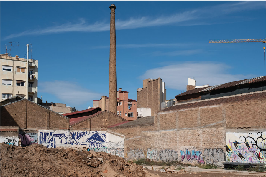
FIGURE 28 Industrial building demolition in Poblenu reveals a listed chimney, 2021.
