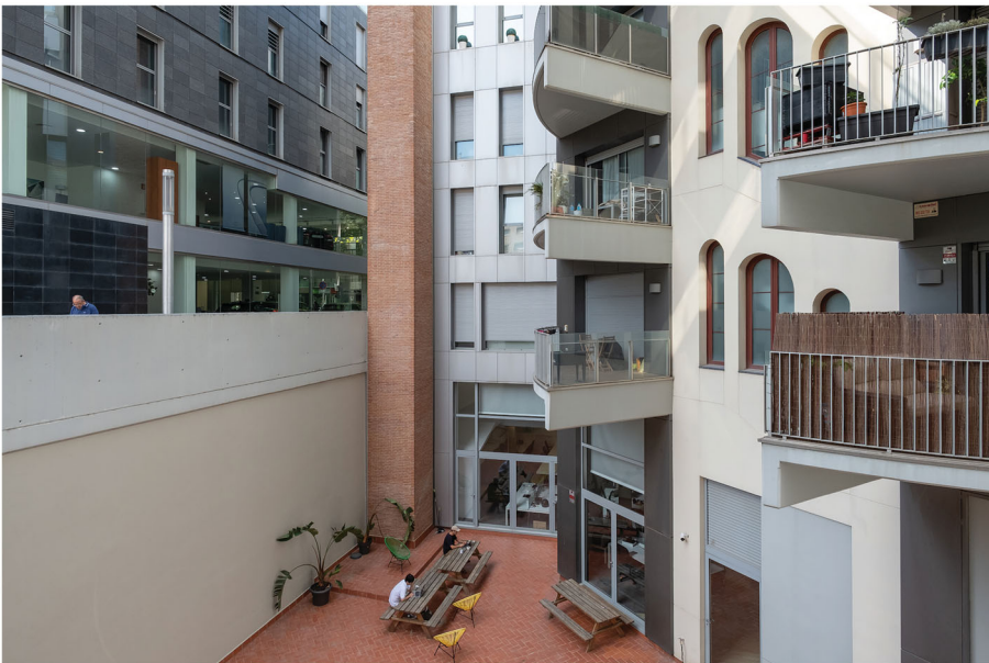
FIGURE 18 The chimney of the Bayer pharmaceutical factory in Eixample. When the factory was closed in 2003, only the factory's façade was retained. The chimney was relocated brick-by-brick, propped by a new luxury residential building, 2021.
