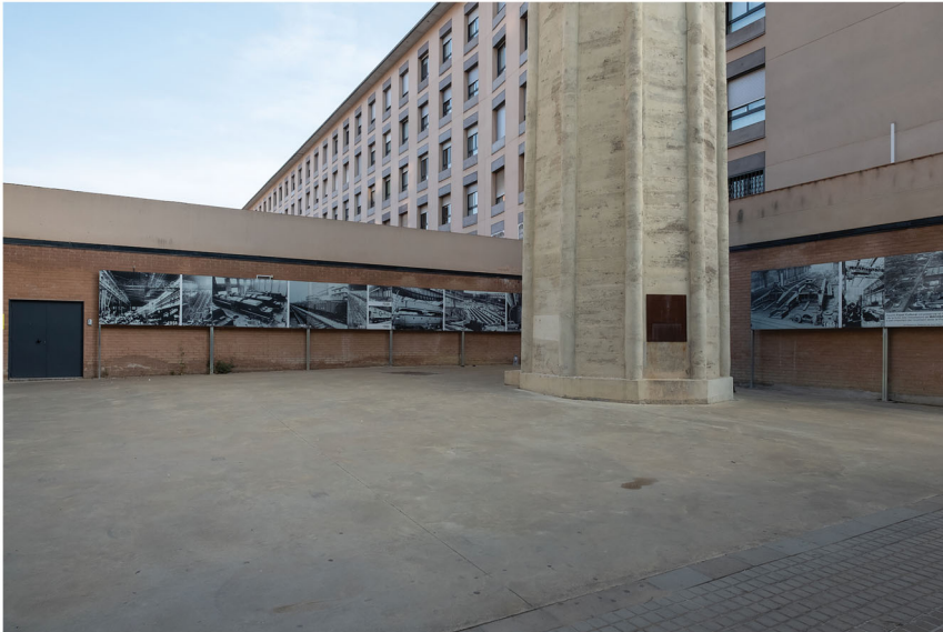
FIGURE 19 The site of the former MACOSA factory in Poble Nou, manufacturing trains until 1991, contains Barcelona’s tallest and most recently built smokestack (1950). It is surrounded by a luxury housing complex. In 2017, after sixteen years of campaigning, retired members of a labor union inaugurated a “memory space” around the chimney, depicting the history of the site, including labor and antifascist struggles and workplace hazards, 2021.
