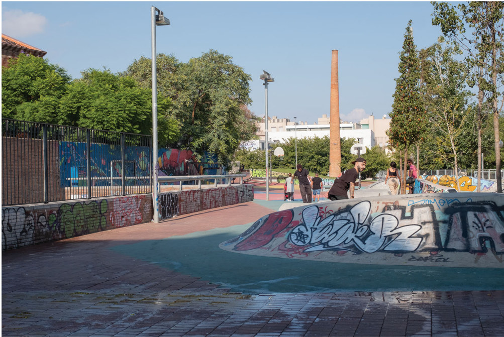
FIGURE 4 This chimney in Jardins de Sant Pau de Camp in El Raval, is one of the three remaining chimneys of the over 300 that once existed in the old, walled city. It was one of the first chimneys to be consciously protected from demolition, around 1980. Like many other parks on former industrial land, the economic viability of the park was justified by the construction of a multi-level parking lot underneath, 2021.
