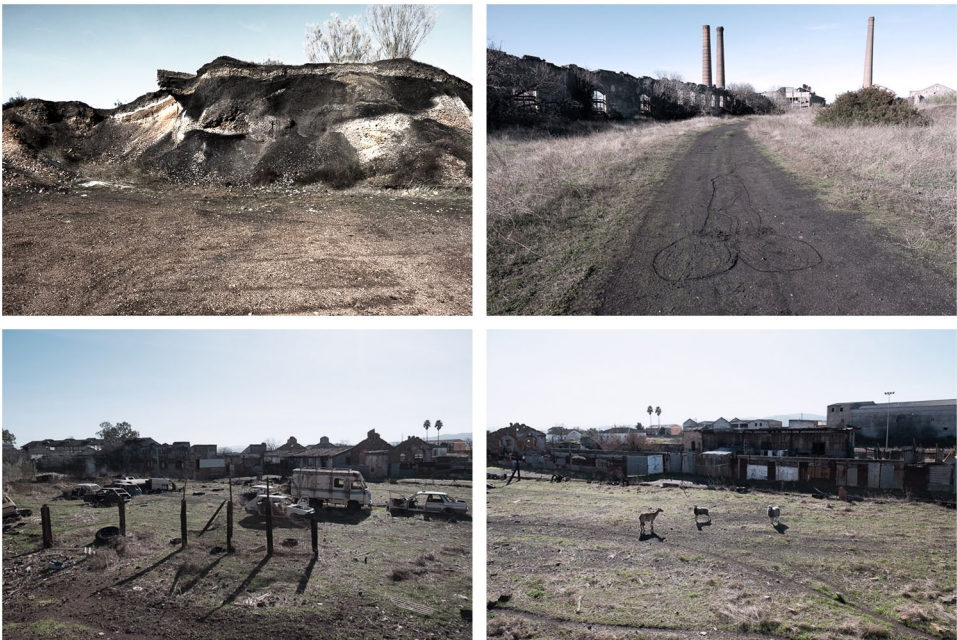
Figure 3. Earthworks and other works (photographs by authors, 2022).
